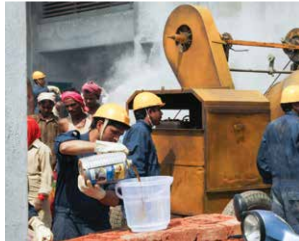
▲ Workers concoct the right mix for waterproofing.
