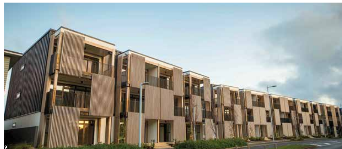
9. The Grounds have Vulcan screening & sand decking as sun shades – made of Abodo wood – from Span Floors.
