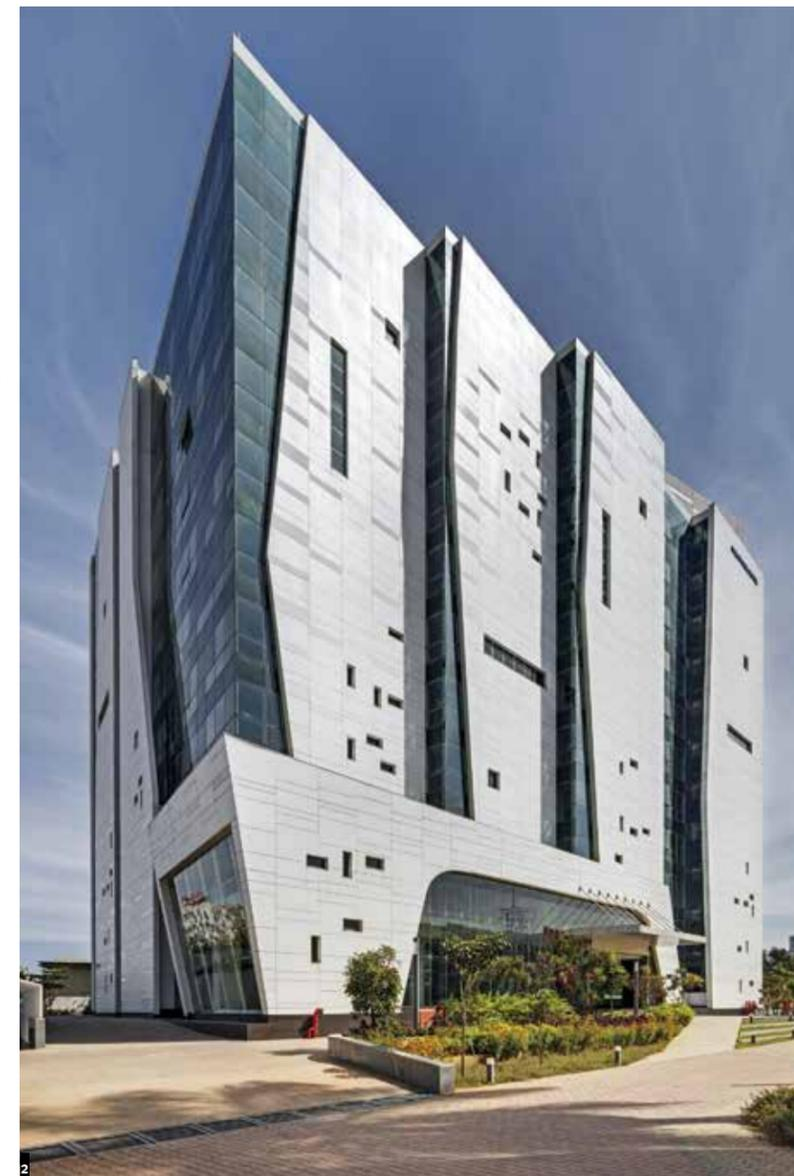
2. FunderMax façade system installed using the rear ventilated principle can be used in combination with other materials in high-rise structures.
