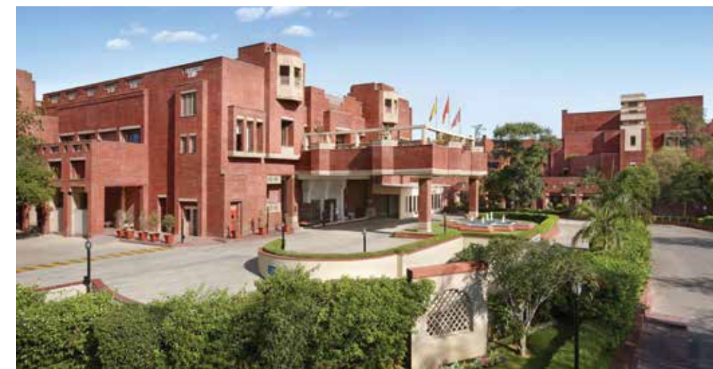
Millennials are deeply aware and choose to stay in sustainably built hotels, such as the ITC Rajputana, which deploy green material and are responsibly maintained with least impact on the environment.
