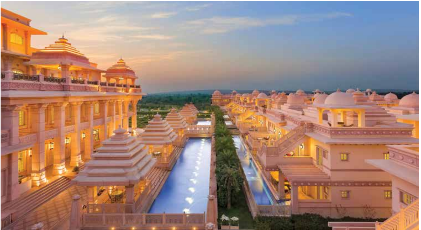
➔ ITC Hotels and Welcomhotels have achieved 100% of 2030 GHG (Green House Gases) emission targets and are in line with COP 21 Paris agreement (66% emission reduction from 2010 base levels).
