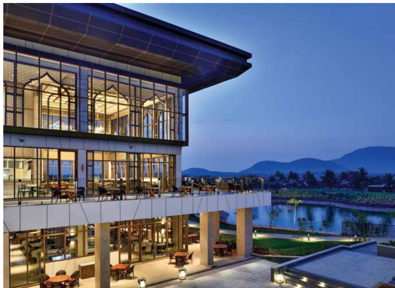
JW Marriott Bengaluru Prestige Golfshire Resort Hotel Hotel & Spa.
