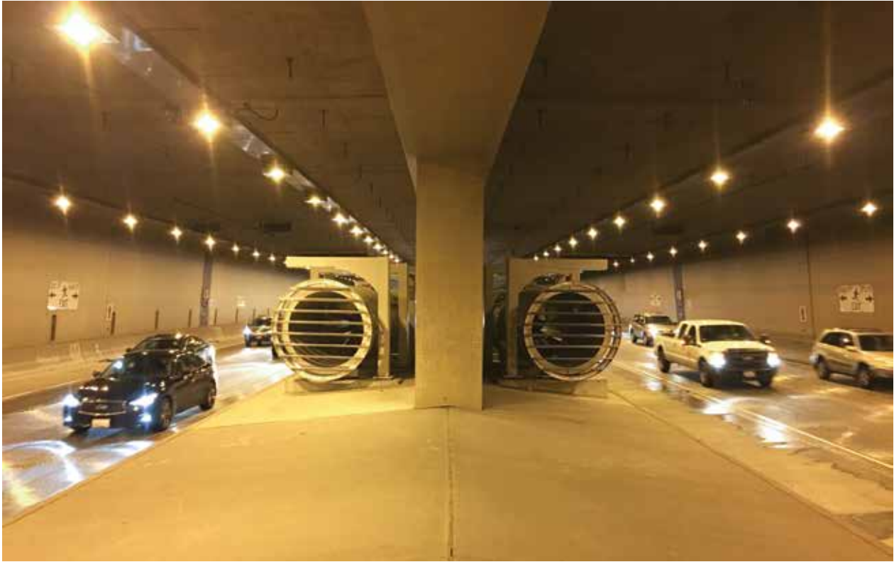
▲ New kinds of blowers keep ventilation going for miles in a tunnel.
