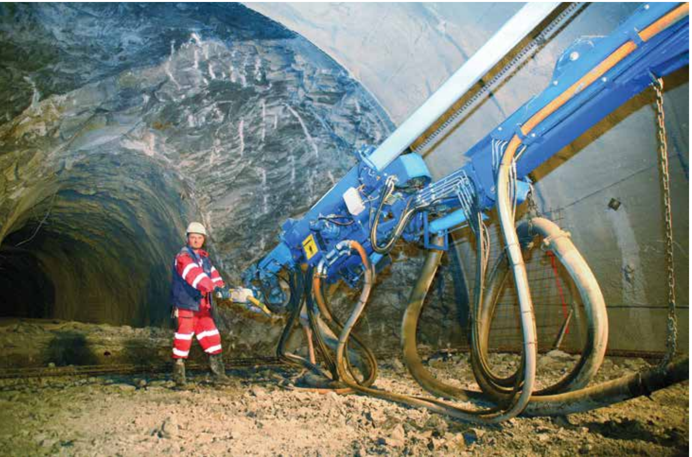
▲ A workman works on a system.
