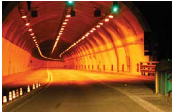
▲ A long view of a tunnel in the Himalayas.
