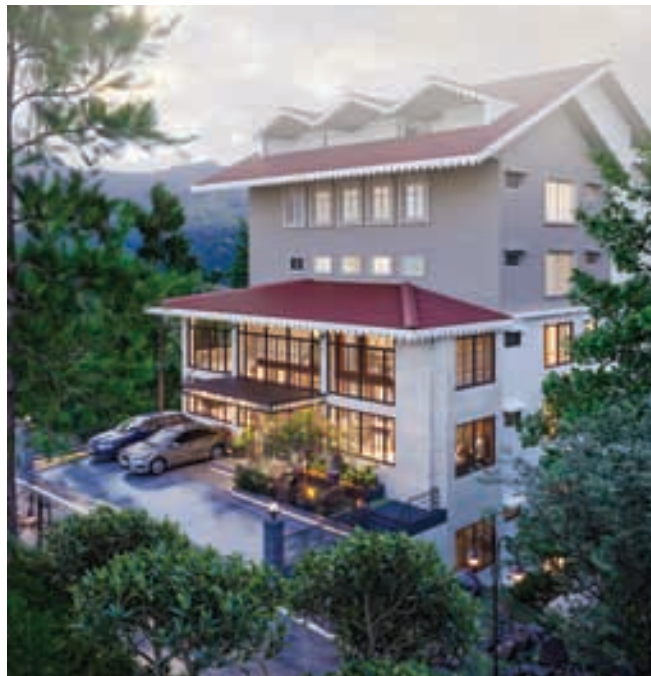
PHOTO COURTESY: 6HUES ARCHITECTURE STUDIO
